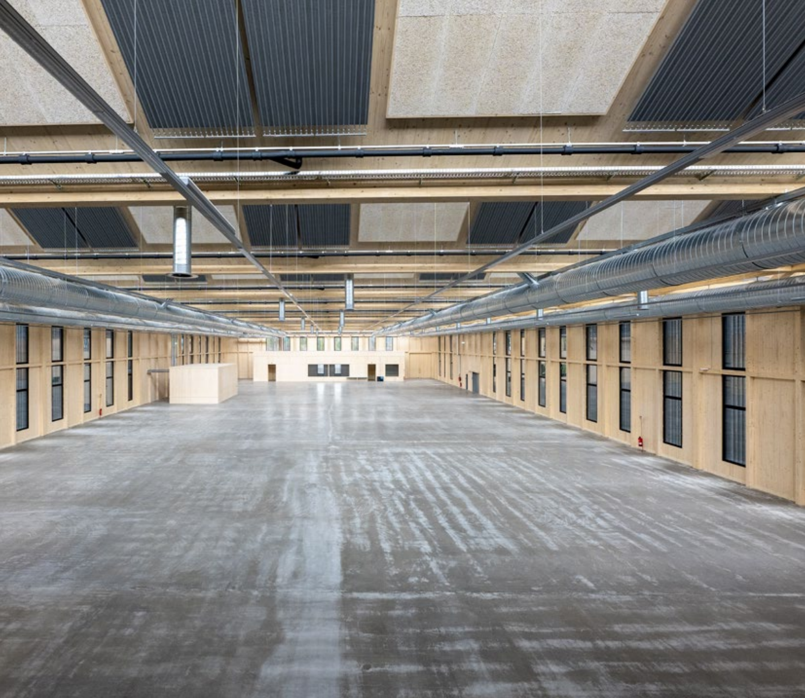
Interior view of the surface technology and toolmaking hall
